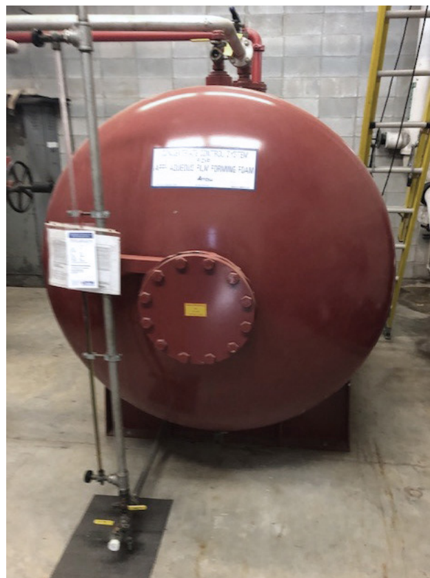
Bladder tank with MILSPEC-compliant (Mil-F-24385) AFFF concentrate
