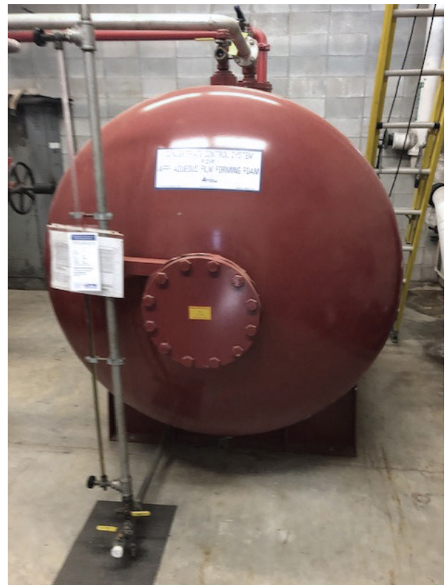
Bladder tank with MILSPEC-compliant (Mil-F-24385) AFFF concentrate
