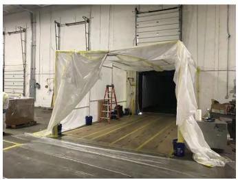
View from the west entrance of the contaminant reduction zone showing the sealed connection to a parked trailer before loading.
