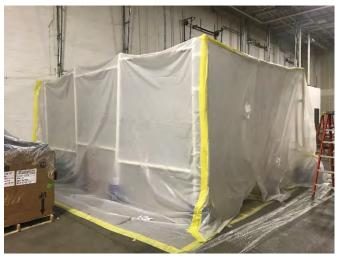
West entrance to the contaminant reduction zone is sealed between shipments when the loading dock is closed.
