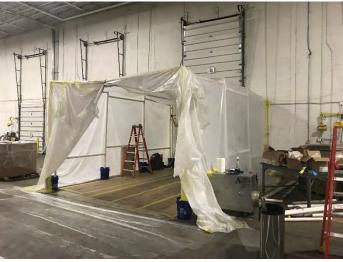
West entrance to the contaminant reduction zone that connects to a loading dock. Negative air machine is on the southwest corner.
