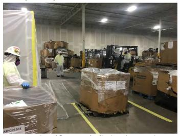
Decontaminated floor space leading into the contaminant reduction zone. Tow-motor was cleaned prior to entering the CRZ.
