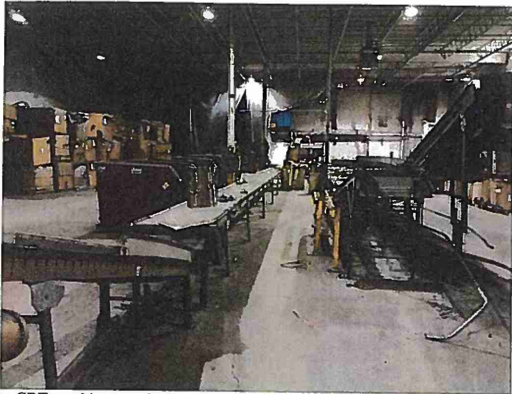
View of the CRT crushing area in the west central portion of building 1675. The CRT crusher is the blue equipment behind plastic sheeting installed as an attempt to control dust.
