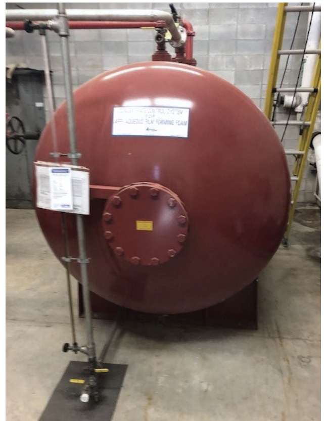
Bladder tank with MILSPEC-compliant (Mil-F-24385) AFFF concentrate
